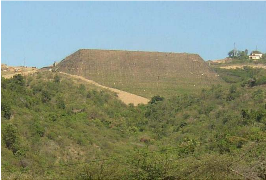
Figure 1: View of the 31.5m high western embankment
