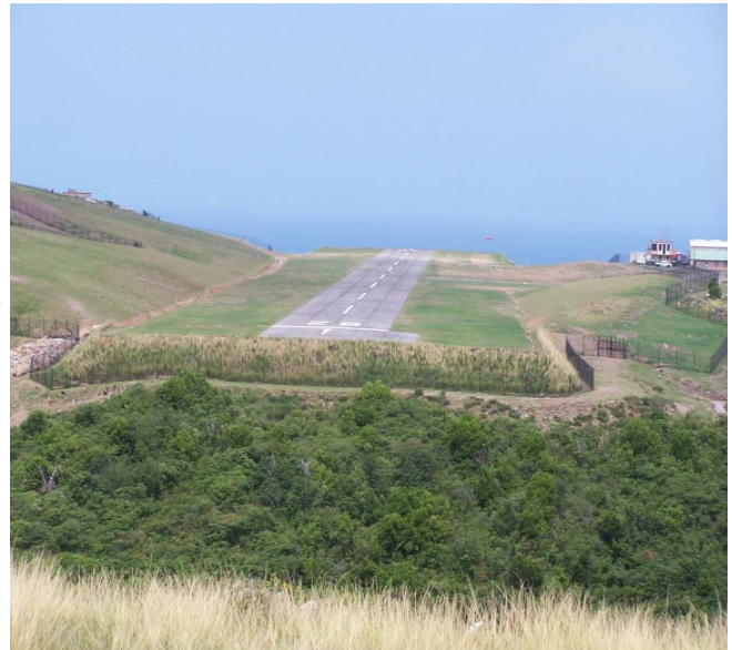
Figure 2: View along the runway from the eastern embankment
